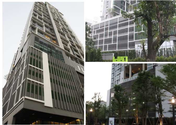
Figure 2 Exterior of the Ideo Mobi Sathorn condominium
